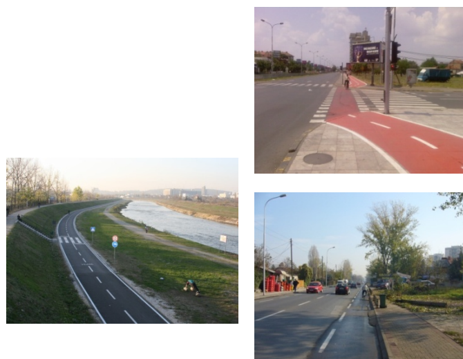
Fig. 2: a) cycling paths b) cycling lanes c) recreational cycling paths along Vardar river
