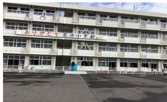
Fig. 1 Arahama Elementary School
