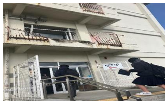
Fig. 2 Exterior wall of Arahama Elementary School
